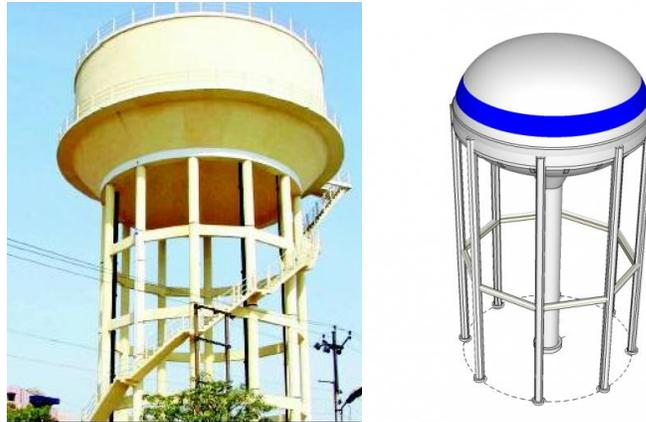
**Figure (d): Intze type Water tank** **Figure (e): Spherical type water tank**
