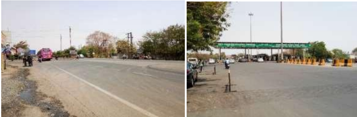
Fig 7. Condition of road on Alwasa Square to Baroli Toll Plaza.
