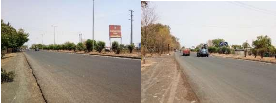
Fig 7. Condition of road in front of Raoti Range (BSF) Training Centre
