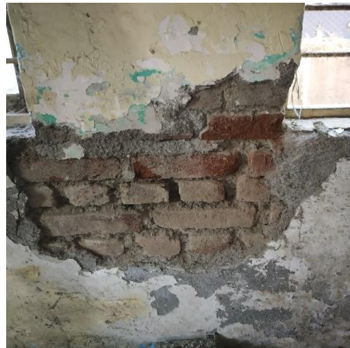
Fig.4 Exposed brickwork
