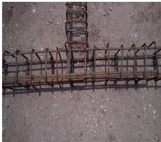
Fig.9 Exterior Beam-Column joint cage
