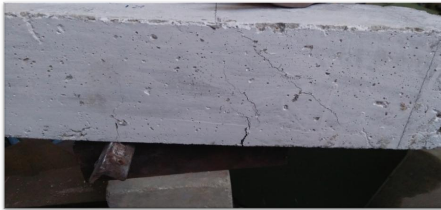
Fig 7. Shear-flexural mode of failure
