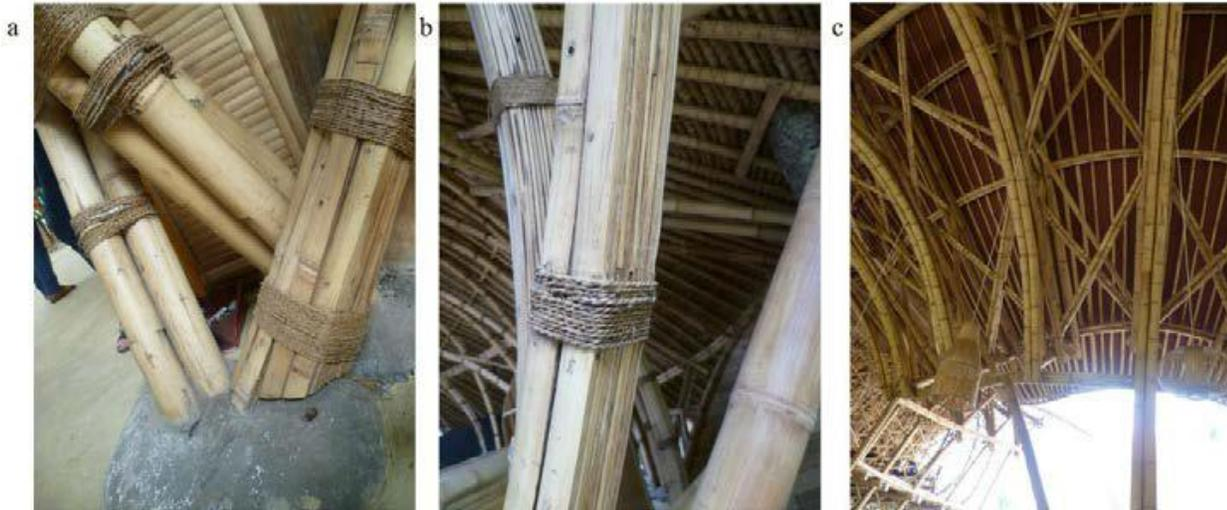
**Fig. 4 Structural details; (a) Bamboo split method and bamboo bundling; (b) Bamboo split details; (c) Detail of arches using bamboo bundling.**
