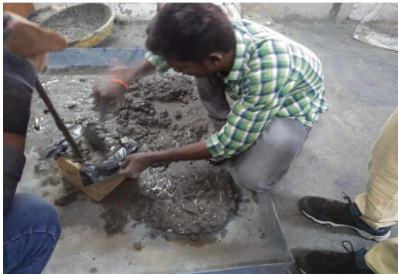
Mixing of concrete
