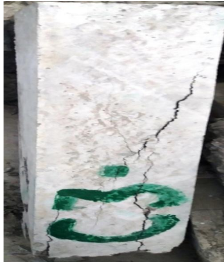
Figure 3 Cracking in Column after compression test
