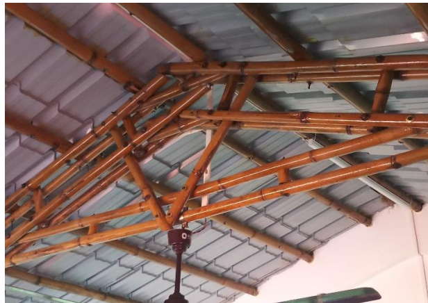
Fig. 3 King's Truss Made from Bamboo
