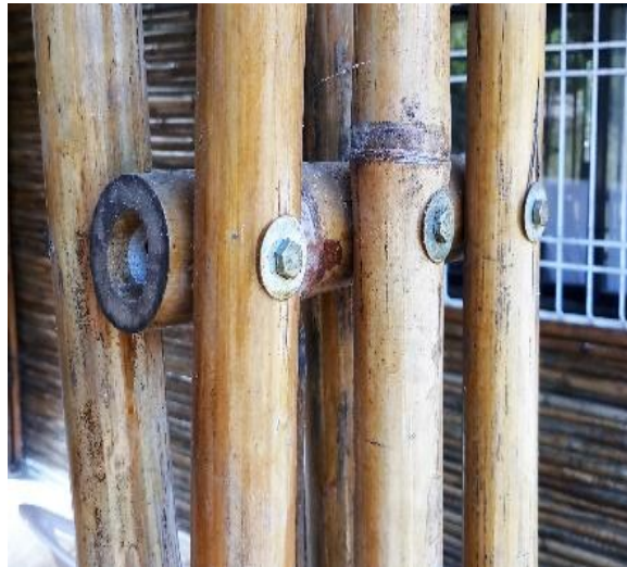
Fig. 2 Joint in Column
