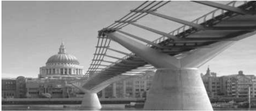
Figure 1 London Millennium Bridge
