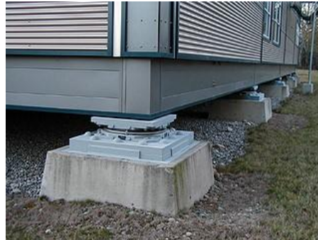
Fig. 1 Friction Pendulum Bearing
