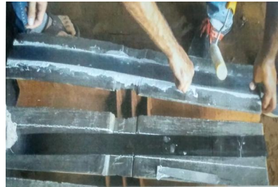
Fig. 10 application of CFRP sheets on steel sections without end anchorage
