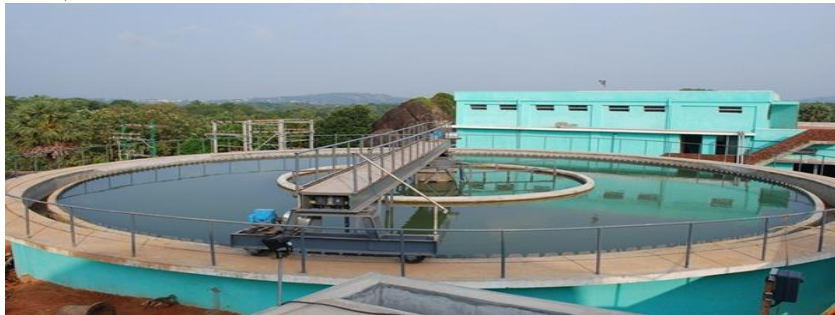
Figure-5- Clariflocculator
