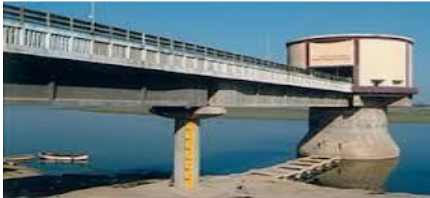
Figure-1-Intake well
