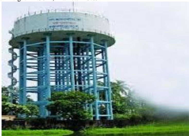
Figure-9- Elevated storage reservoir
