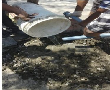
Fig 2: Mixing of Concrete
