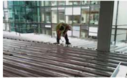
Fig 2: Composite deck slab
