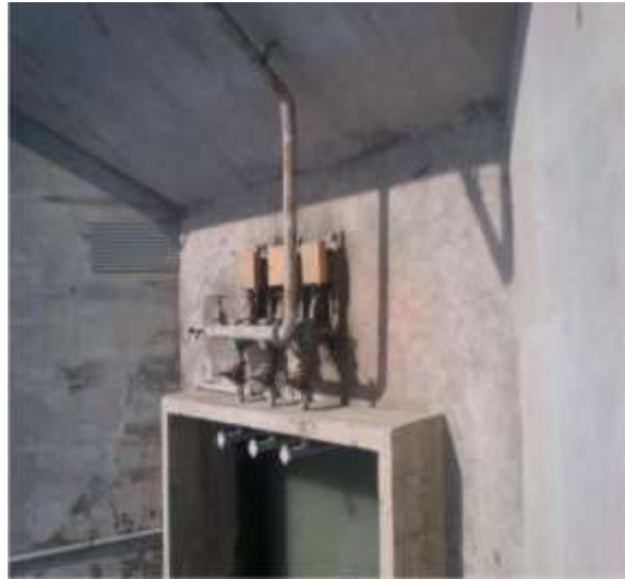
Fig.2. Raw Sewage Pumps
