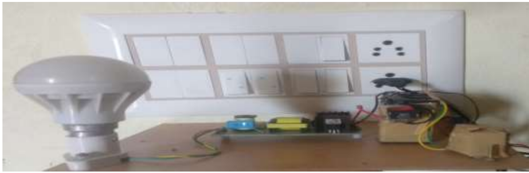
Fig.4. Power supply charging the battery
