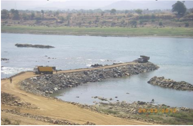
Fig. 5 Under construction Garudeshwar weir site
