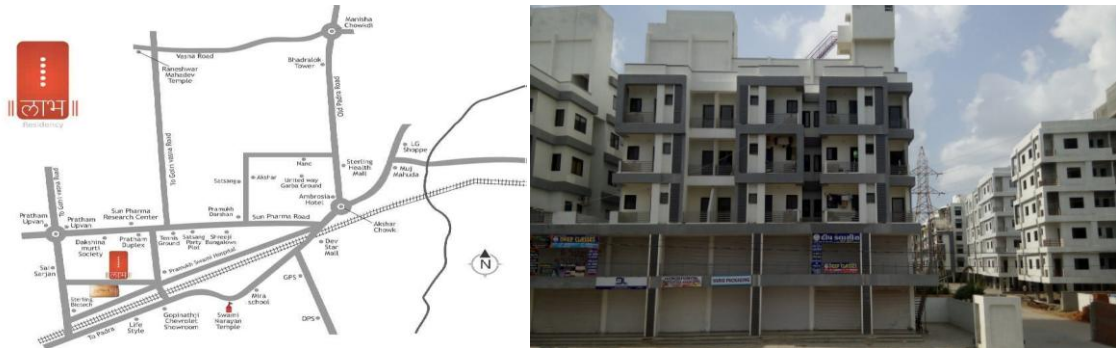
Fig. 1 layout & Photographic view of Low-rise Building
