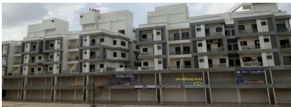
Figure.5. Front View of Tower No.13 A &B
