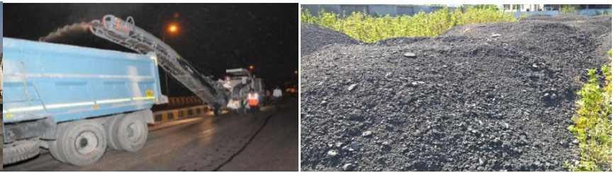
Figure 2: Material Stockpiled at Surat
