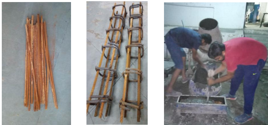
Fig. 2 Re-bar and Beam Casting
