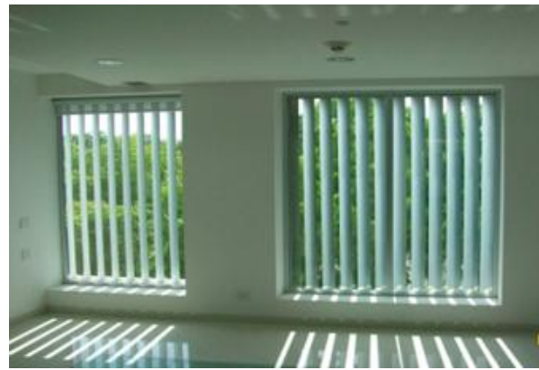
A. Day lighting (Outside view with Glare control with window to wall ratio: 0.48)
