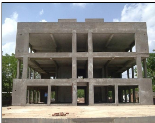
Fig 2 A. Existing unused structure
