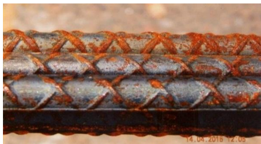
(c) : Fresh ribbed TMT bars showing start of corrosion at ribs (three days after ribbed bars reached the construction site)
