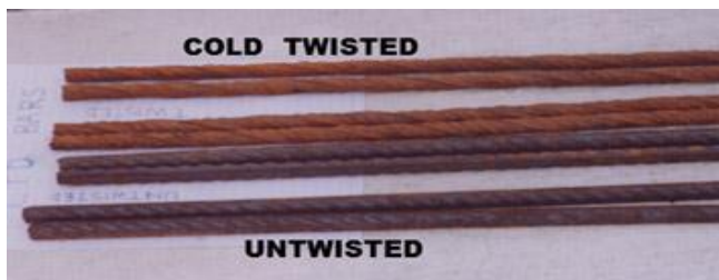
(a) : Rebars with ribs showing start of corrosion preferentially at the ribs of untwisted bars (four bottom bars) and corrosion all over the surface when the remaining length of the same bar was twisted beyond yield at a cold state (four top bars) (CTD bars)
