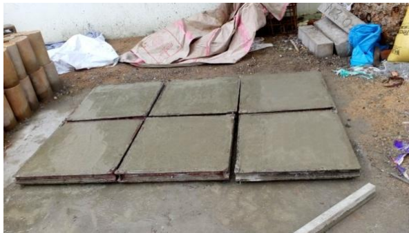
Plate 5: Casting of slabs of 600x600x50mm
