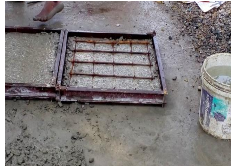
Plate 4: Slab mould with reinforcement
