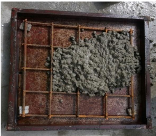
Plate 3: slab mould with reinforcement
