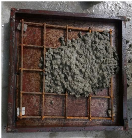
Fig 3: Slab mould with reinforcement
