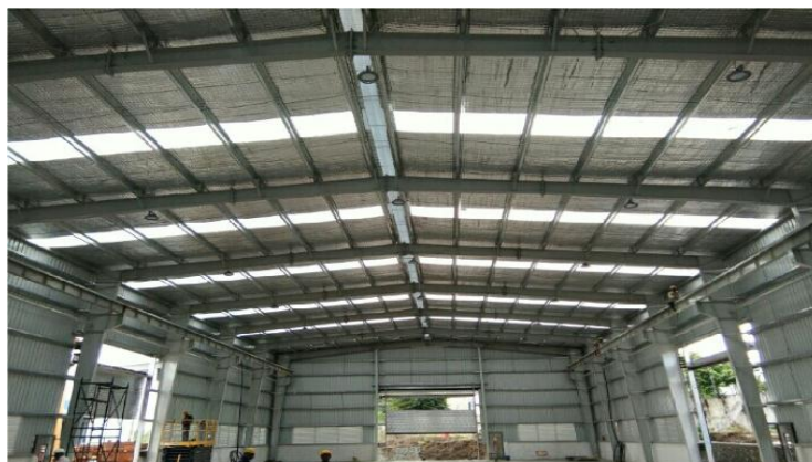
Fig. 1: Pre-Engineered Warehouse Structure
