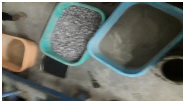
Fig:2 Materials for concrete Mix
