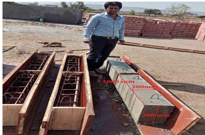
Figure 3.1 - Moulds with casted Beam
