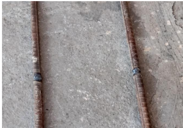
Figure.1.2 - Butt Welded splices
