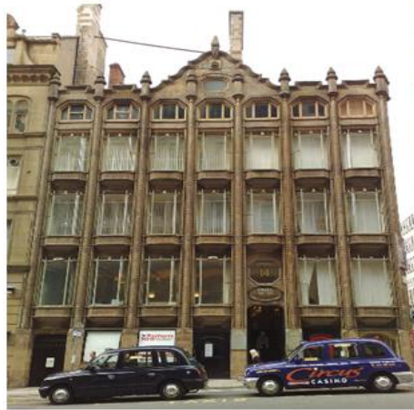
Fig 1: Oriel Chambers, Liverpool. The world's first glass curtain walled building.
