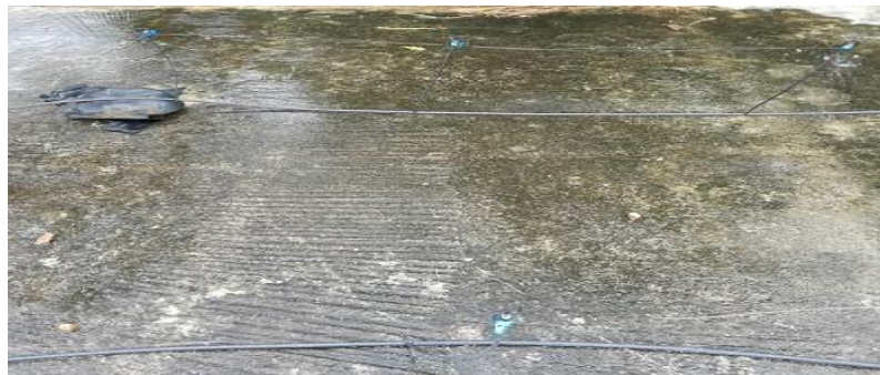
Fig.3 Water sprayer's arrangement on roof of case study building
