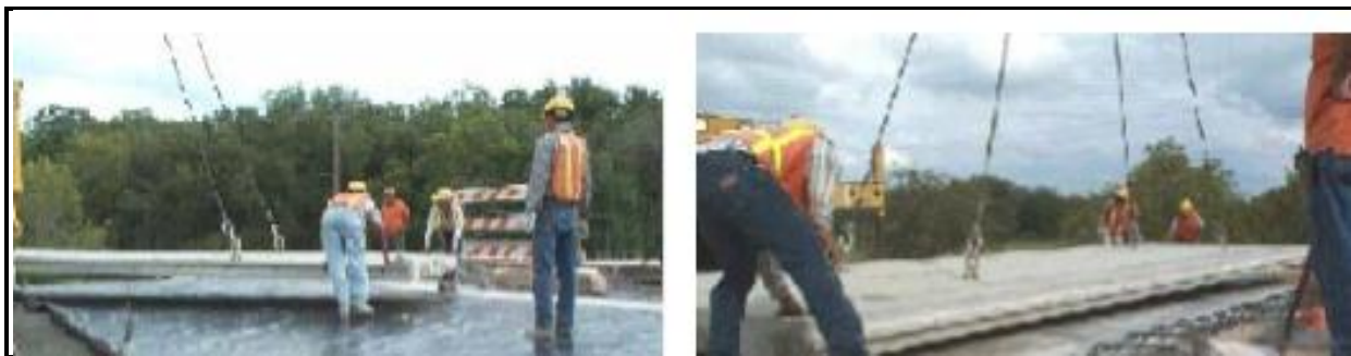
Fig 3.7 (a) Place Polyethylene Sheet
