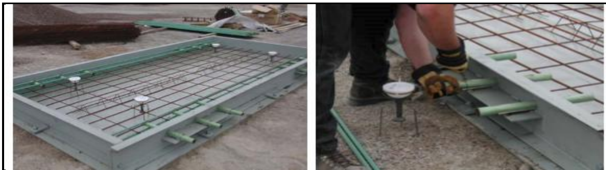
Fig 3.2 Reinforcement and Dowel Bar Placement in the Formwork
