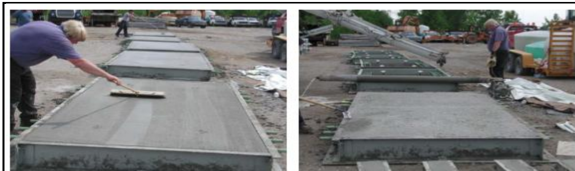
Fig 3.3(a) Concrete Placement
