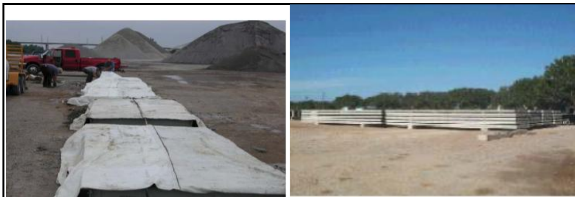
Fig 3.4 (a) Curing of Precast Slabs
