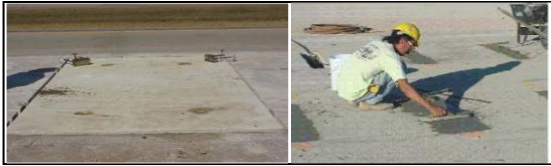
Fig 3.9 (a) Stabilized Slab
