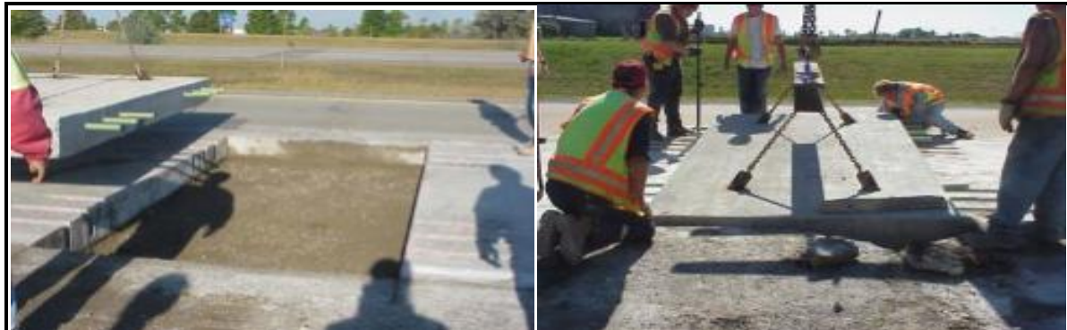
Fig 3.7 (a) Place Polyethylene Sheet
