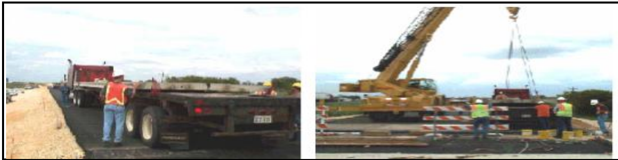
Fig 3.6 Transport Panels to Worksite
