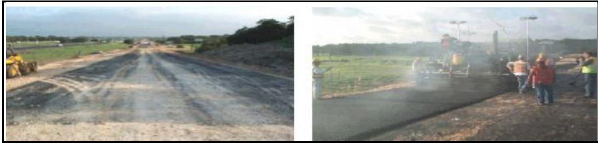
Fig 3.5(a) Preparing Sub-base
