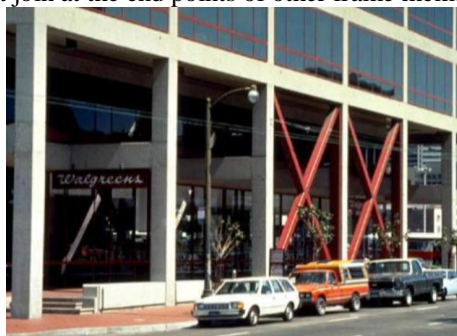
Fig. 1.1 Concentric Bracing
