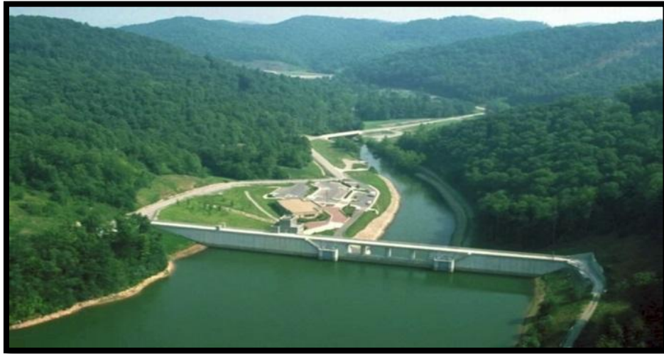
Fig 5: Reservoir on the upstream side of the dam
