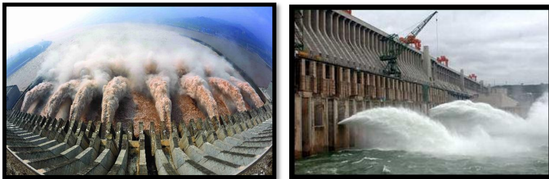
Fig 3: Removal of excess water during floods
