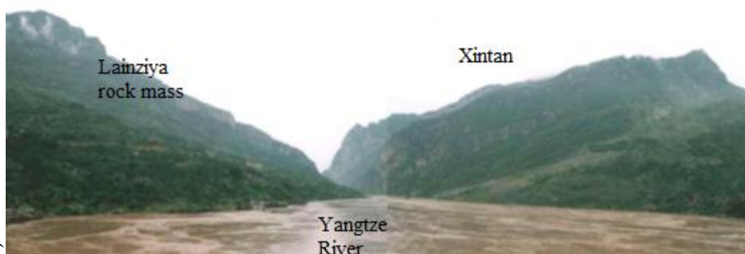
Fig 5: Landslide prone area along Yangtze River
