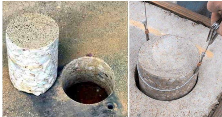
Figure: Core testing of concrete (Source: theconstructor.org)
