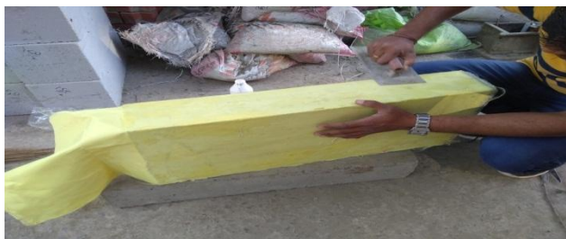
Figure 3 single layer of aramid fiber
