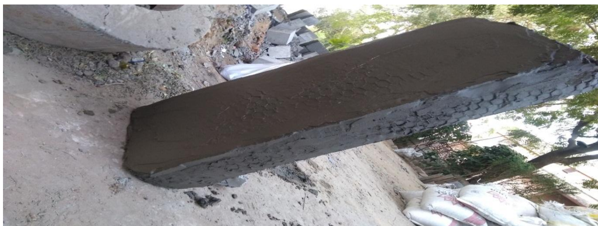
Figure 8 applying cement mortar of (1:3) on Ferro mesh
