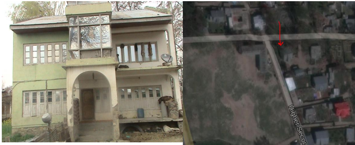
Figure 2: photograph of building (left) and the location of the building on the google map
