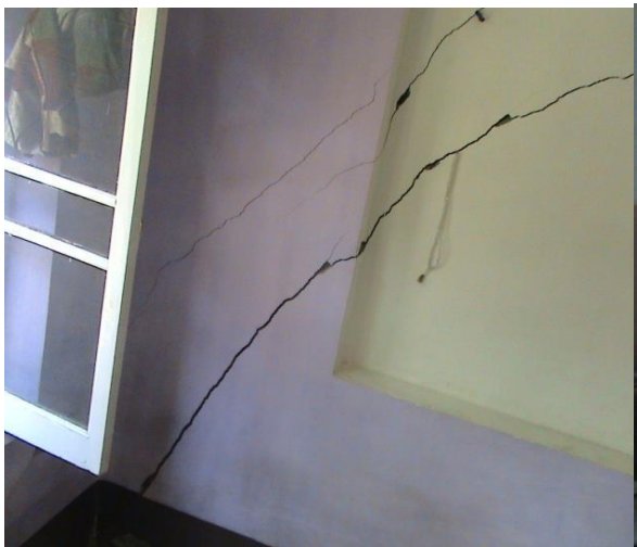
Figure 7: Crack 4( first Floor)
