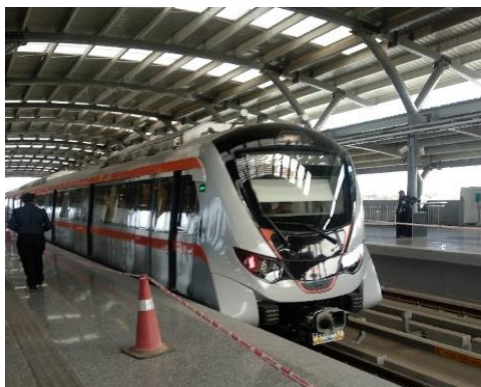
Figure 1 (A) Ahmedabad metro rail
