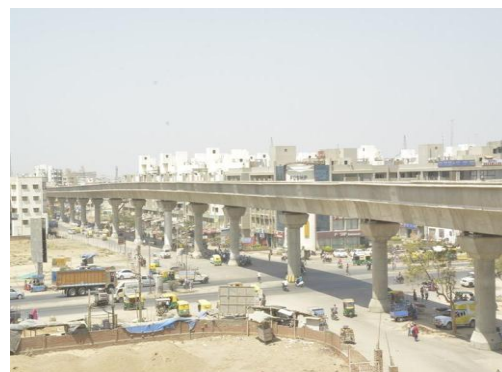
Figure 1 (B) Elevated section of metro rail
