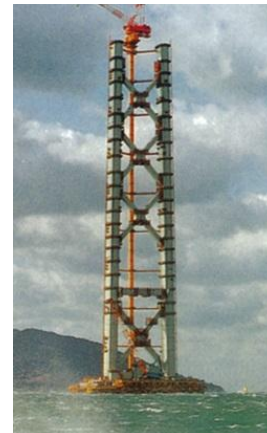
Fig 7: Main tower of the Bridge
