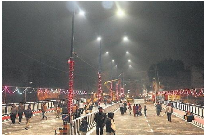
Fig 9: Bridge work completed
