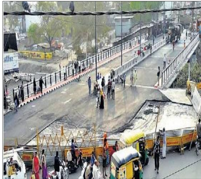
Fig.7 Construction running at the day
