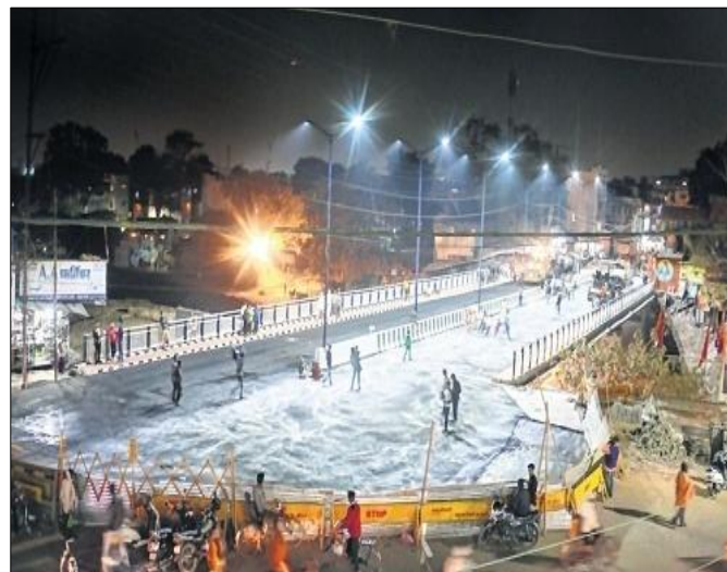
Fig. 8 Construction running at the night
