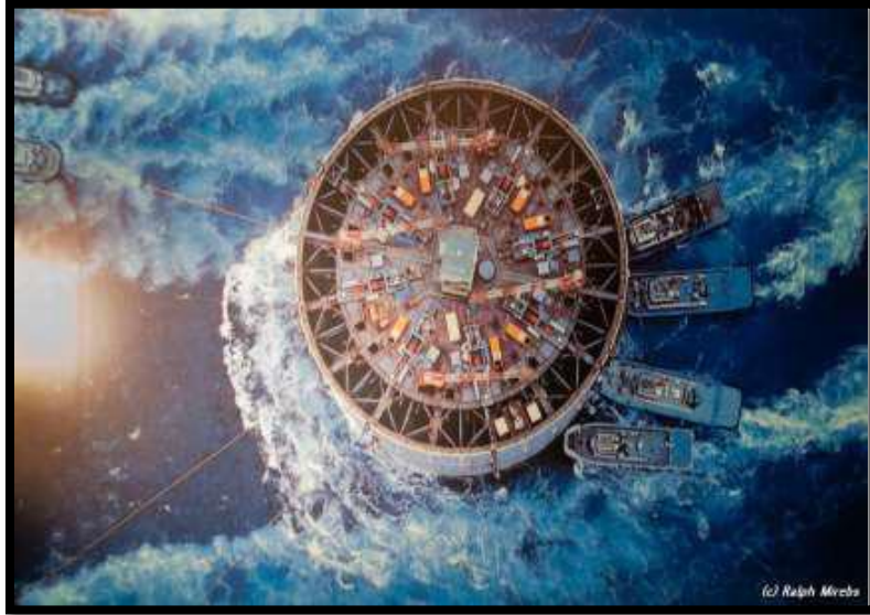
Fig 4: Sinking Of Caisson
