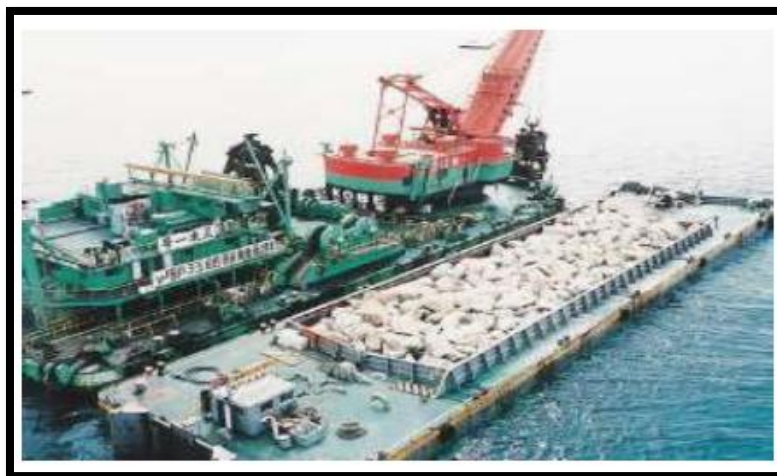
Fig 3: Protection of the Caisson against Scouring
