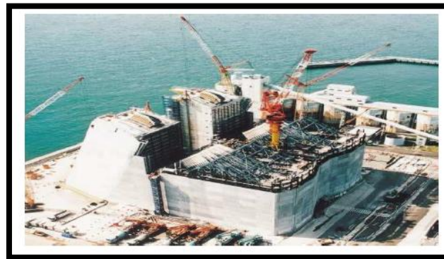
Fig 10 : Construction of Anchorage
