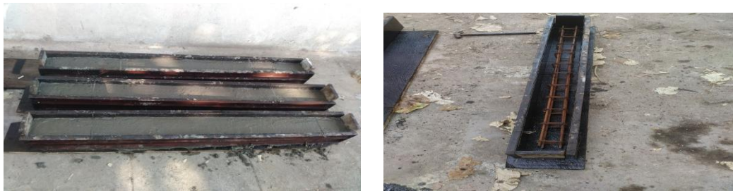
Fig. 3 Casting of columns
