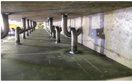
Fig.5 J-hook Connectors in SCS Sandwich System
