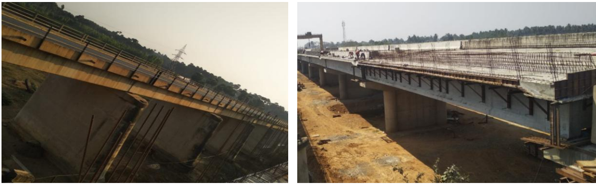
Figure1: Old Bridge and New Bridge at site
