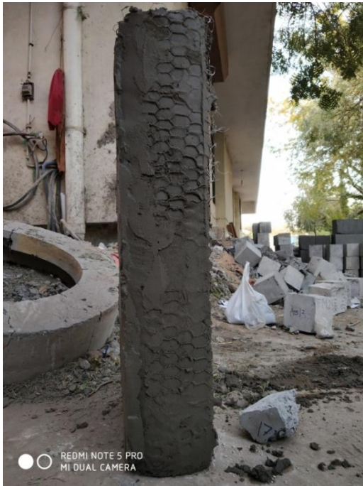
Figure 6 applying cement mortar of (1:3) on Ferro mesh
