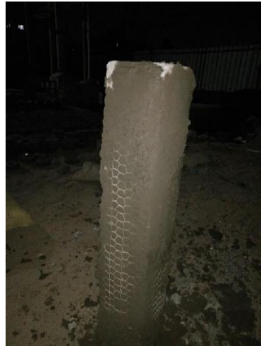
Figure 7 applying cement mortar of (1:3) on Ferro mesh
