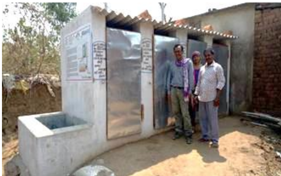
Bio-Toilet (#4) in Pandaripani Village in Kanker
