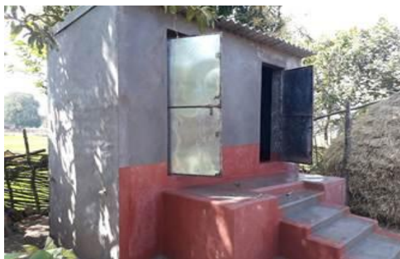
EcoSan Toilets (#2) in Sonpur Village in Kanker
