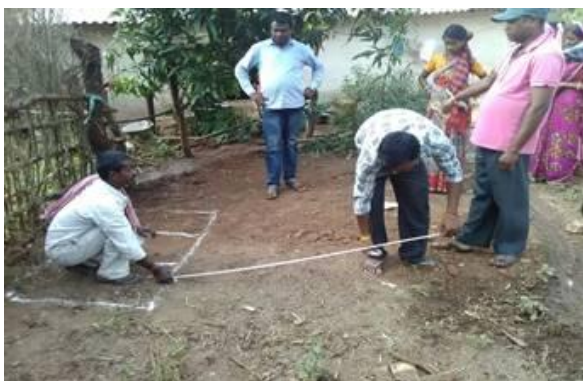
On site training of masons on construction of bio-toilet
