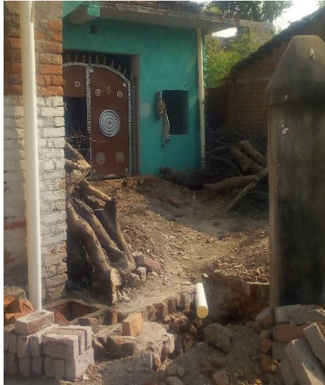
Pipes connected in one end with roof and other with chamber
