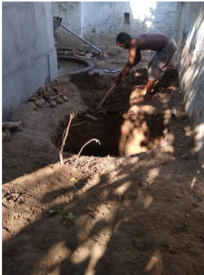
Digging of recharge pit nearby India Mark II handpump
