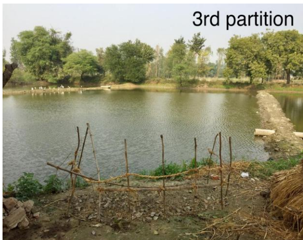
Figure 5: Waste Stabilisation Pond (WSP) in Lalpur: Anaerobic Tank, Facultative tank, maturation tank and clear water tank
