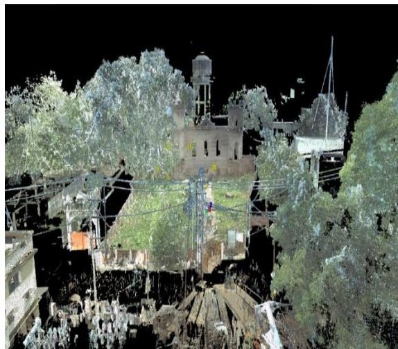
Figure 1 Point Cloud Data of Alambagh Gate with the location of TLS scanner points (before classification).
